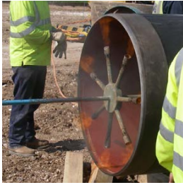
Figure 2. Preheating of pipe end with 'spider' flame torch arrangement.
