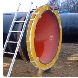
Figure 3. Preheating of pipe end with induction heating coil.
