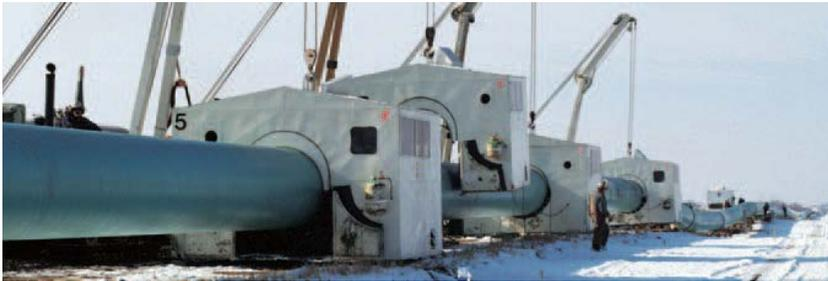
Figure 1. Typical field welding station for automatic welding.
