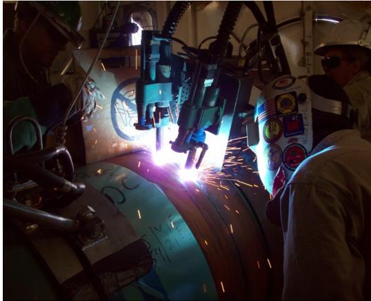
Figure 8. Application of dual torch pulsed GMAW on North Central Corridor.
