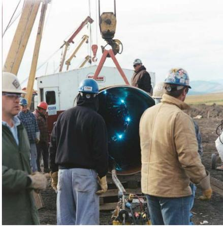
Figure 4. Westpath, internal welding of the Gr. 690 using the 4 head, short circuit GMAW.
