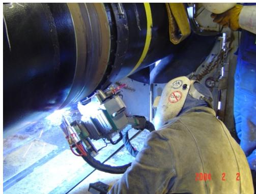
Figure 6. Application of single tandem on welding Gr. 690 Godin Lake.
