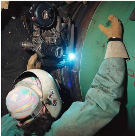
Figure 5. Westpath, external welding of Gr. 690 using the single arc pulsed GMAW procedures.
