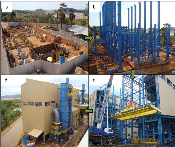
Figure 4. Sinter Plant II; (a) Construction site and foundation, (b) View of columns and beams, (c) Lift crane installation, (d) Sinter Plant II general view.
