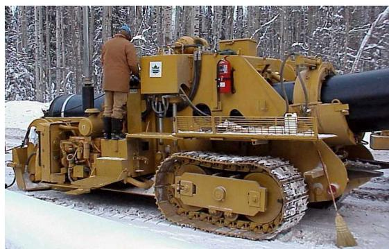
**Figure 20. View of field bend of X120.**
