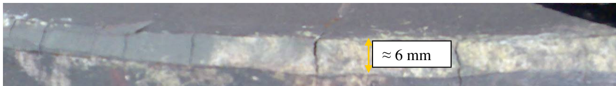
Figure 3: Cracks at corners of rings forged to final shape.
