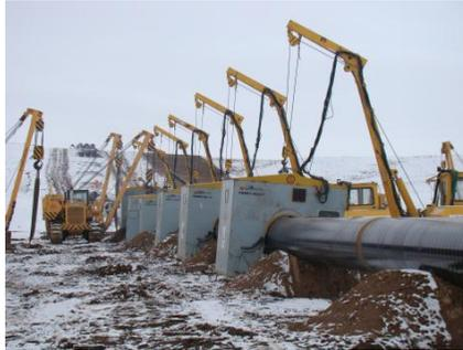
Figure 13. Construction arrangement for the automatic welding group.
