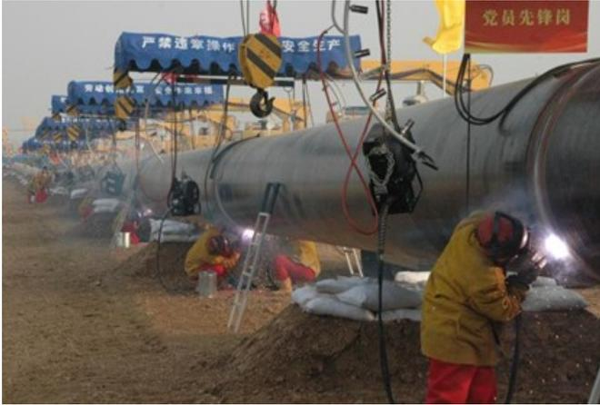
Figure 17. Construction arrangement for the semi-automatic welding group.
