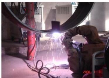
Figure 4. Self-shielded flux-cored wire semi-automatic welding PQR.
