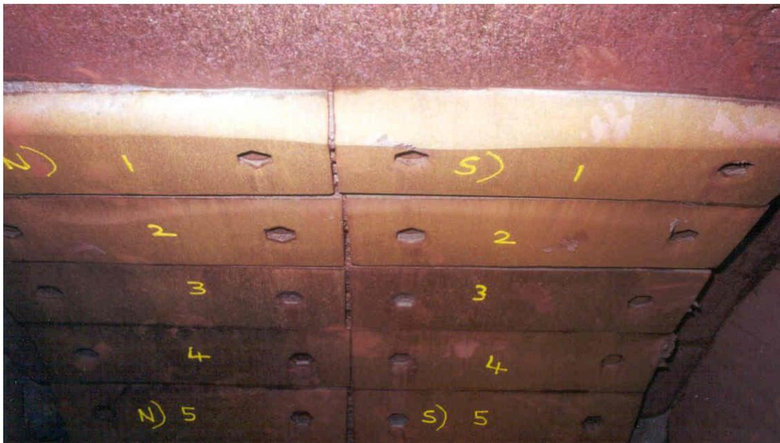
Figure 8. Retrofitted NiHard 4 cast liner segments bolted to the original continuous lining in the upper “hood” section of a live chute in Port Hedland, Australia. The added plates were not sufficient to span the whole of the impingement zone at the entrance to the hood.
