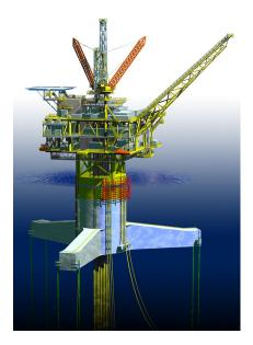
Figure 1. Principle of a TLP (the Atlantia Offshore Sea Star Design)
