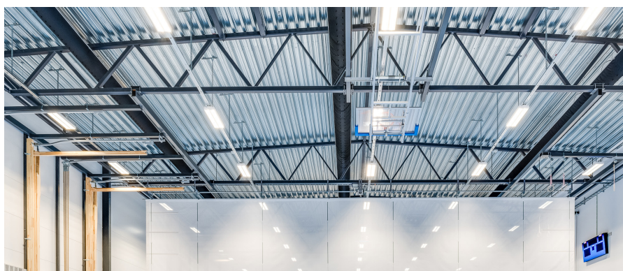
Figure 4 Main arena columns and roof trusses Courtesy: Svante Lundbäck SE
