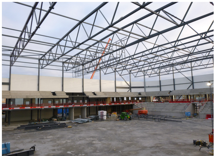
Figure 5 Main arena roof trusses spanning 52 m being installed Courtesy: Ruukki
