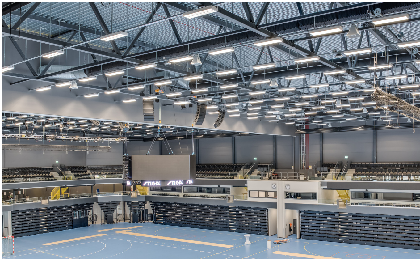
Figure 3 Main arena roof trusses Courtesy: Svante Lundbäck SE
